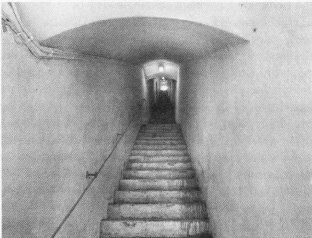
Roedean Tunnel - Photo by Nick Catford
